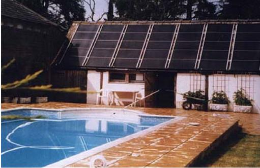
This is almost identical to mounting the panels on to a bank, i.e. instead of sloping earth we have sloping tiles or slates.
