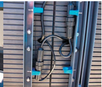
Units are linked electronically and locked mechanically
