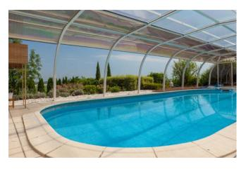
The high-strength profile system used in Aquacomet Endless Summer enclosures creates an opportunity to enclose wider pools. Fixed load bearing profiles are installed every 2 meters, while transparent, solid polycarbonate glazed doors between the profiles easily slide up to provide access to the pool. In this way the enclosure can be opened up to a height of 2.2 m along both sides. The segments are split horizontally into two parts and these 1.1 m parts
