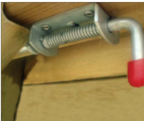
STEP 83 - Lean the steps against the pool with the eyes under the 96 x 96 horizontal timber. Screw on the two spring bolts so as the bolt passes through the eye when the bolts are in the closed position.
