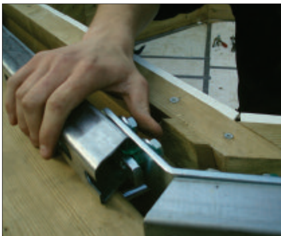
STEP 35 - Insert bracket into next length of steel. Push up to meet the corner and tighten the bolts with the 17mm spanner.
