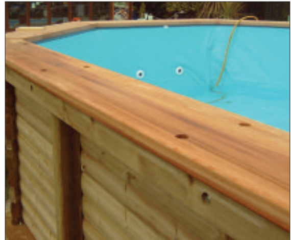
STEP 74 - While the pool is filling with water, place the timber top surround into position around the pool.
