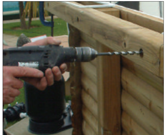
STEP 28 - Drill holes through the timber and pool wall and insert a 230mm x 12mm bolt through from the inside as shown.
