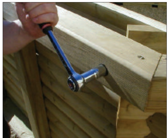
STEP 30 - Using the socket wrench firm up the nuts making sure that the washer is underneath. Do Not tighten fully at this stage.
