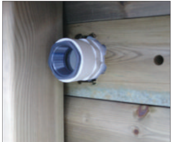
STEP 64 - Glue grey PVC fittings into white fitting using glue provided
