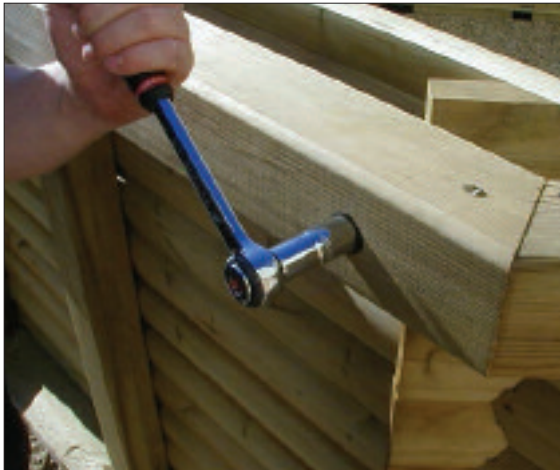
STEP 73 - Go around the pool gently tightening the nuts and checking that the pool timbers are level. Do Not over tighten.
