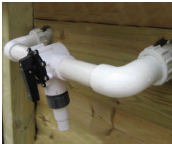
STEP 21 - Attach the return inlet pipe and valve section to the threaded unions protruding through the pool wall. Please note: Make sure 'O' rings are seated correctly inside the unions.
