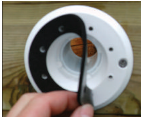
STEP 20 - Make sure gaskets have been fitted and holes are aligned.
