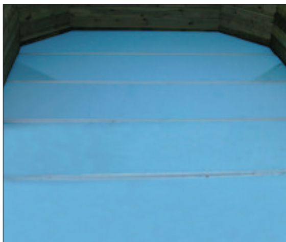
STEP 45 - Fit the pre-cut Styrofoam base and tape the joints.
