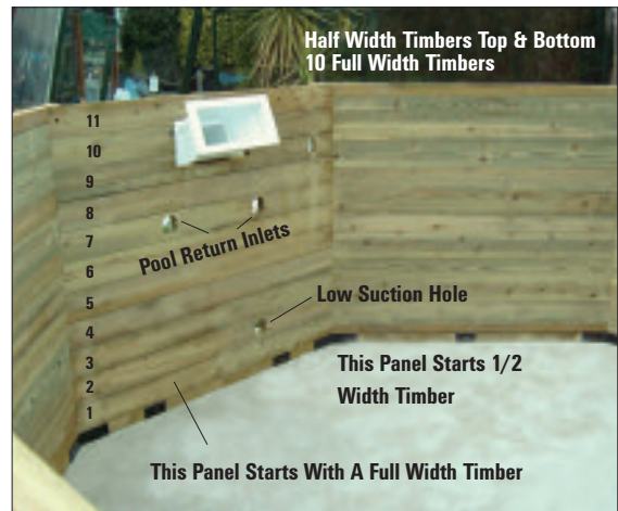
STEP 16 - Where the skimmer is located on a corner wall the low suction is sited at 2.5 log and the returns are positioned at 6.5 log. The skimmer is 9.5 - 10.5 logs. See appendix A / B on page 20.
