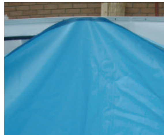
STEP 52 - Start placing the liner in the top groove of the plastic liner-lock. Start from a corner and work your way round.
