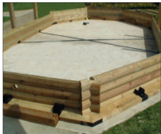
STEP 12 - Continue assembling the wall timbers, alternately aligning the corner joints. Make sure the tongues and grooves are in line before tapping down.
