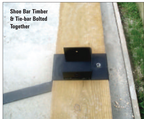
STEP 6 - Line up the shoe and tie bar. Fit the coach bolt from underneath and secure with a nut and washer.
