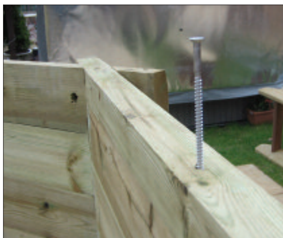
STEP 23 - Screw the half timbers to the top of the pool wall with the 100mm stainless steel screws.
