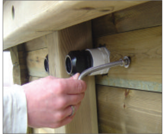
STEP 68 - Push threaded rods through the hole, leave nut and washer on the rod, cut a small incision in the liner for the rod to go through.
