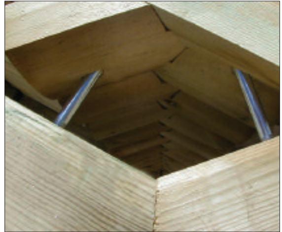
STEP 32 - View of the two corner bolts from above.
