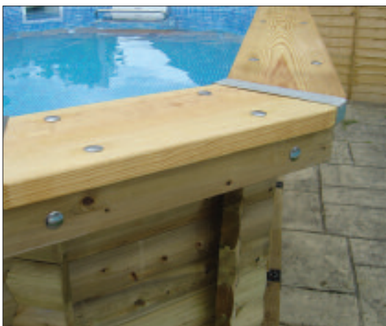
STEP 75 - Line up all 8 corners with an even overlap of the timber. Make use of the clamps to help hold the timbers into position. Also using straps as per step 31 will make the process easier.
