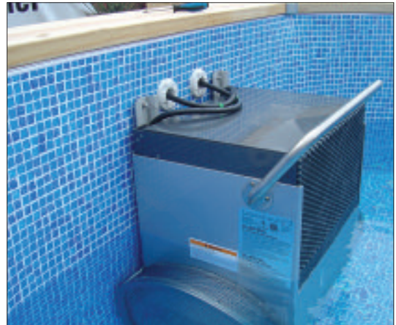
STEP 70 - Thread the hose through the Fast Lane fittings.
