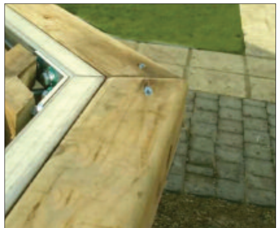
STEP 36 - The steel ring beam should lay tightly inside the timber ring beam all the way around the pool.
