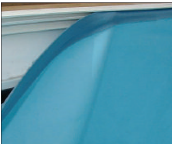
STEP 53 - Push the top of the liner into the top groove of the liner-lock.
