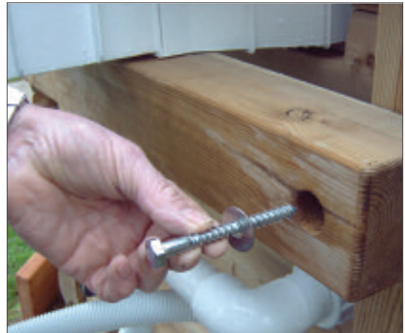
STEP 40 - Hold the skimmer support timber under the skimmer. Using the 100mm coach screws and washers, tighten with the socket wrench so that the timber supports the skimmer.
