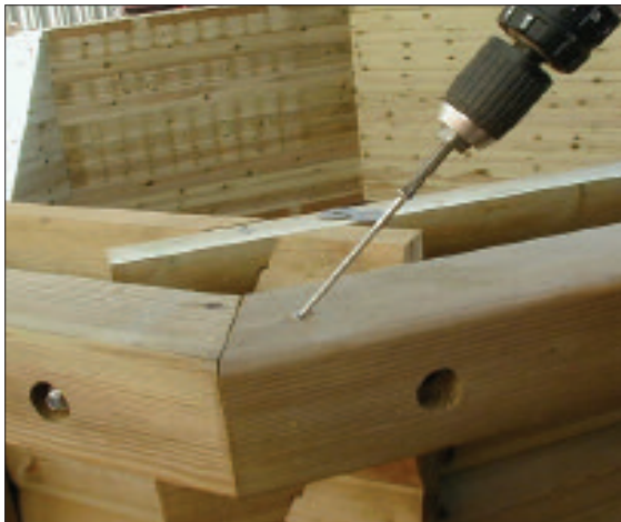
STEP 33 - Align the corners and insert the 100mm stainless steel screws as shown top and bottom making sure that the corners are aligned and level.
