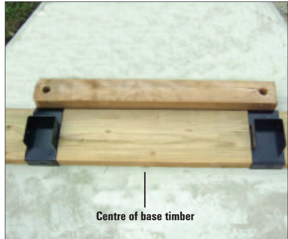
STEP 8 -The skimmer panel has two steel shoes. Use the skimmer support timber to help centre and position the steel shoes. Do not fix at this stage.
