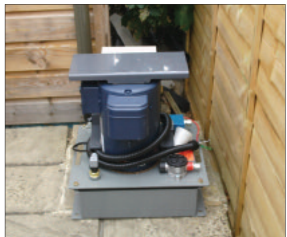
STEP 72 - Attach the hose ends to the hydraulic pump (hose ends are colour coded). Refer to the Fast Lane manual for the start up procedure.
