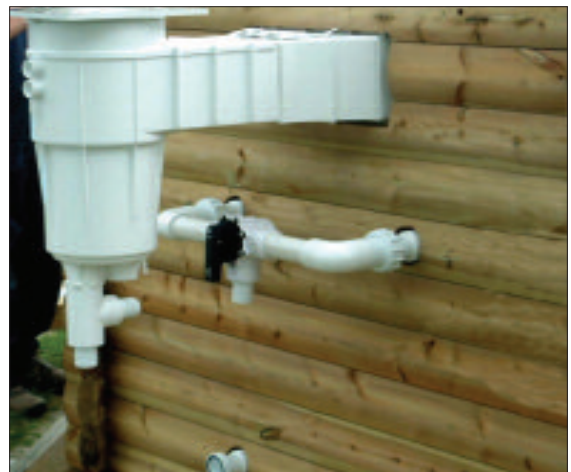
STEP 22 - The skimmer, return inlet and low suction in position. Viewed from the outside.
