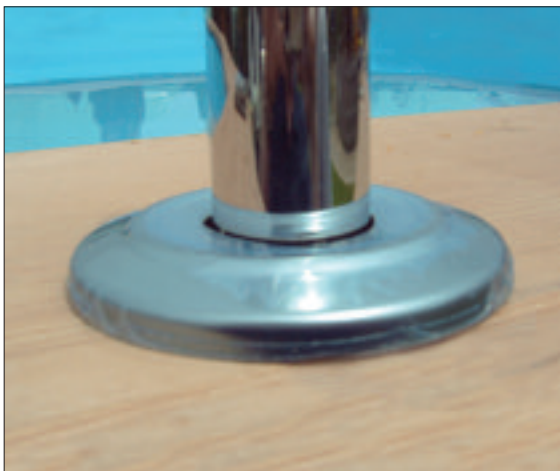
STEP 81 - Place the stainless steel covers and then assemble and fit the steps. Assembly instructions for the steps are in the steps box.
