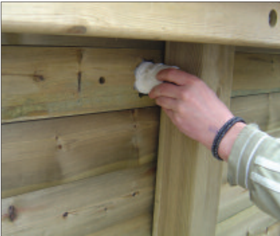
STEP 63 - Silicone white fitting in to the Fast Lane fitting
