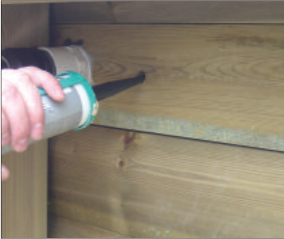
STEP 67 - Squirt silicone into the hole for threaded rods
