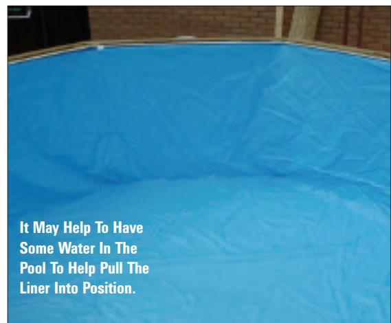
STEP 54 - Continue pushing the liner into the liner-lock all around the pool and then push out the creases with your feet. Do Not wear shoes for this procedure.
