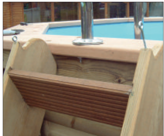
STEP 82 - Screw in the two eye screws into the top of the underside of the wooden pool steps as shown above.
