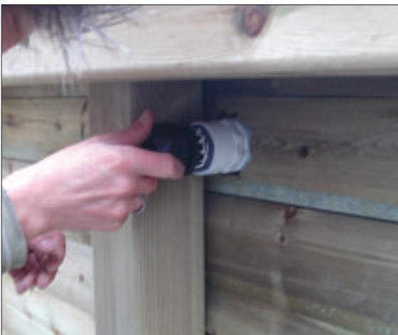
STEP 65 - Silicone black Fast Lane fitting into the PVC fitting
