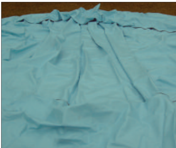
STEP 51 - Lay the liner in the pool as close to the position that the liner will be finally fitted. The liner is shaped to fit the pool, so make sure it's the correct way around. Take off your shoes when working with the liner otherwise you will mark it.
