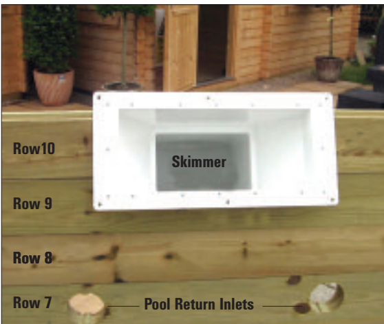
STEP 15 - Rest the skimmer on this aperture before fitting the top timber.
