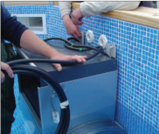
STEP 69 - Lower the Fast Lane into the pool and attach to the rods with the remaining nuts and washers and tighten.
