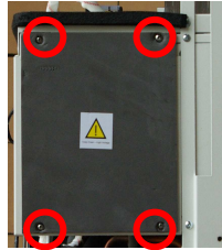
Open the electrical compartment
