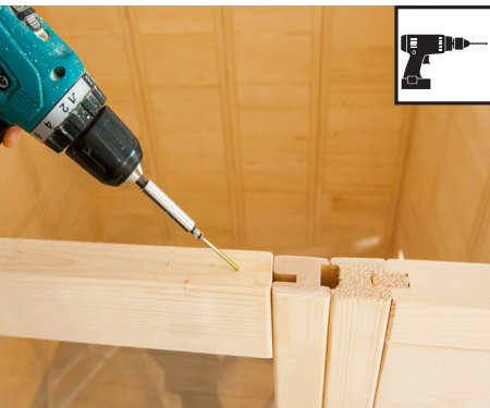
Foret de 3 mm, 1 vis 4 x 70 mm
