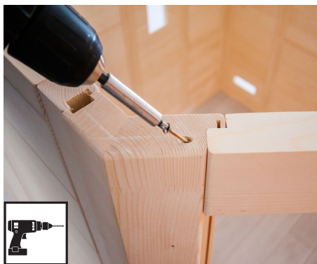
Foret de 3 mm, 1 vis 4 x 70 mm
