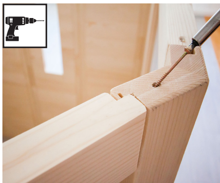
Foret de 3 mm, 1 vis 4 x 70 mm
