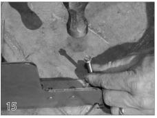
Use the 1 1/2 hex head screws (26) and anchors (25) provided to secure the motor end and non motor end to the deck.
