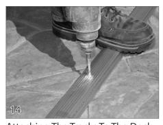
Attaching The Tracks To The Deck Place the Tracks into position on the deck in the marked positions. Make sure that the tracks run completely straight on both sides of the pool. Drill through the pre-drilled track holes into the deck. Drill at least 3" deep.
