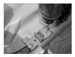
Install a stop on the end of the track near the mechanism to keep the cover from retracting too far. Secure the stop to the deck using the screws (15) and anchors (25) provided. Run the key switch in the uncover position to roll the cover up on the roll-up tube. Check the cover to be sure it rolls up evenly.
