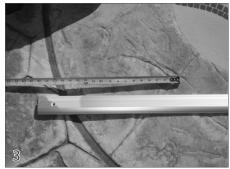
Extend the tracks at least 18" past waterline. Center the pool shape between the pool tracks where possible. Measure and mark the track space and track length on the deck.
