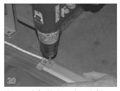
Place a guide feed (14) over the end of the track and drill 3/16 hole through the hole in the guide feed and through the track.
