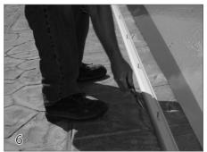
Feed the rope into the back channel then pull the rope down the back side of the track toward the cover housing.
