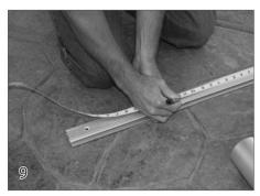
Cutting The Tracks To Length With the track extended at least 18" past the waterline at the opposite end of the pool, cut the tracks so they extend 18" past the waterline at the mechanism end.
