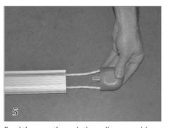
Feed the rope through the pulley assembly (17) and insert the pulley housing into the end of the track.
