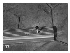
Place the track back over the holes in the deck. Fasten the track screws (15) <u>halfway</u> through the tracks into the plastic anchors. The screws will be fastened completely later in the installation.
