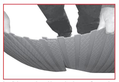
Install the second panel by overlapping onto first panel as shown.
