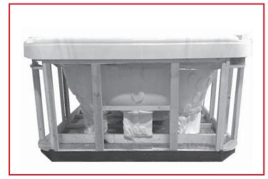
If not already framed in, use a couple of 2x4's to frame out an opening for an equipment service panel. The service panel should be at least 24" in width, but can be wider. A third 2x4 will be used as a horizontal support. It needs to be installed as a backer to fasten the service panel to.
