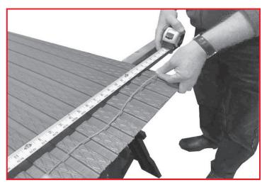
Measure the length of one of the spa panels and cut a piece of string to the exact length. The string will be used to layout the panels around the spa.
