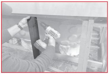
Add additional bracing if necessary, bracing should be no more than 24" apart.
