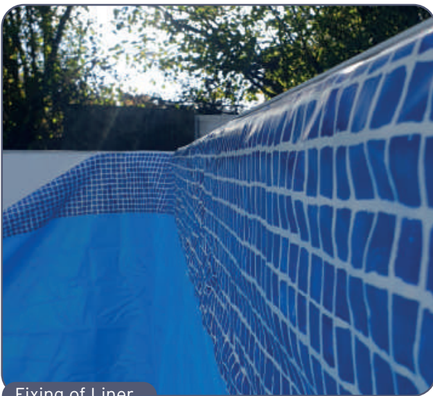
Fixing of Liner
