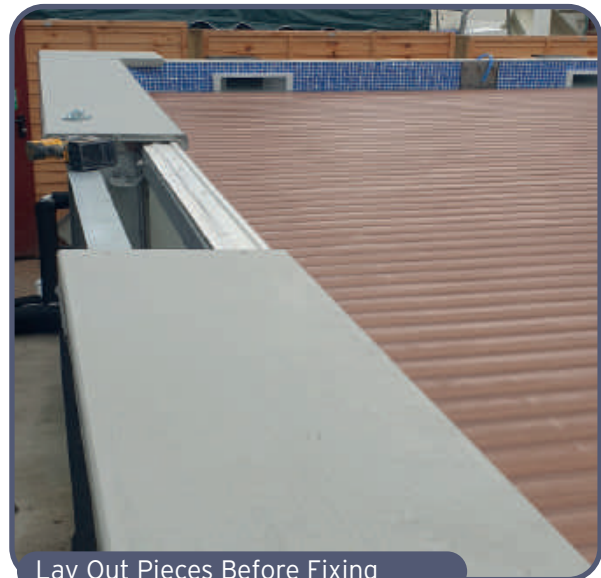
Lay Out Pieces Before Fixing
