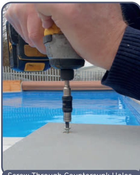
Screw Through Countersunk Holes
