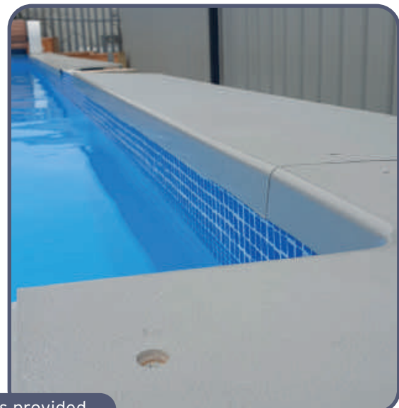
Lay Out Pieces Before Fixing
