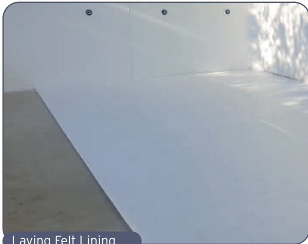
Laying Felt Lining
