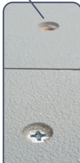
Cap off screws with caps provided
