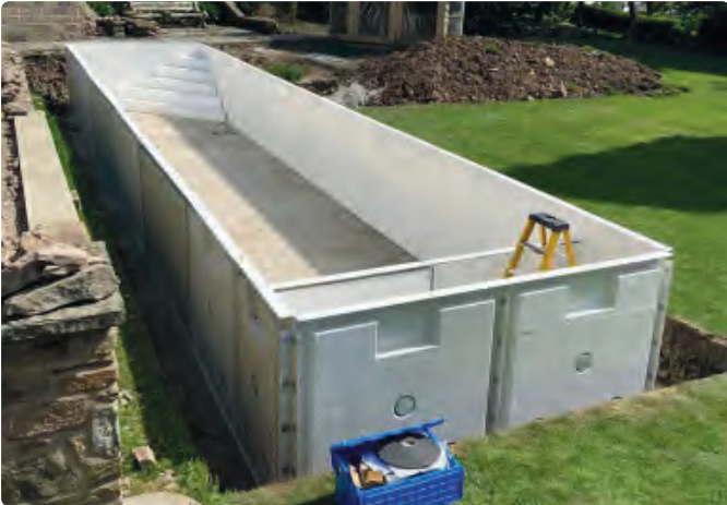
Above: Pool shell constructed within a day.
