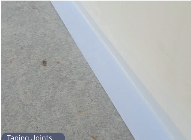
Taping Joints
