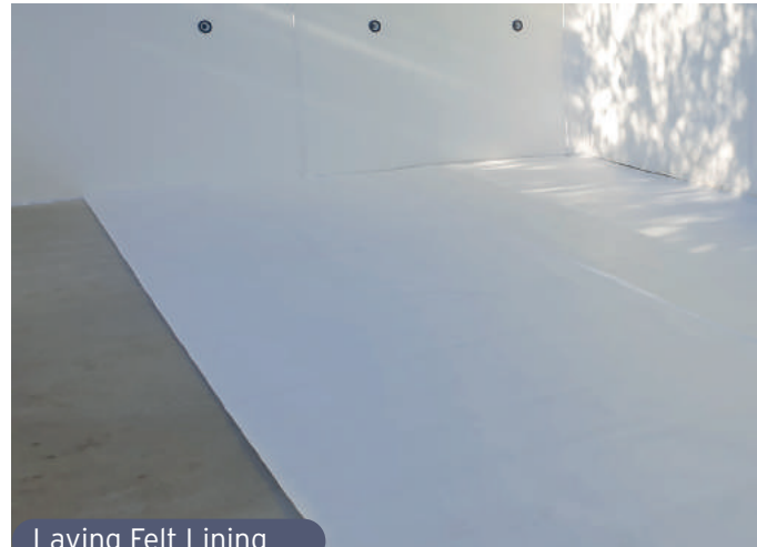
Laying Felt Lining
