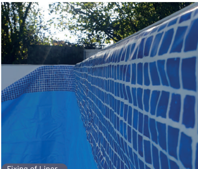
Fixing of Liner
