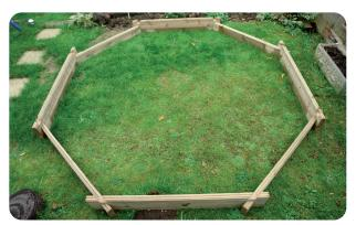
Using 4 standard planks you can now form the first layer of the pool walls. The 45 degree interlocking slot at each plank end will form the shape of your pool.
