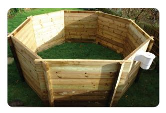
The next stage is to insert your top full planks and upper skimmer plank. These have two grooves and a flat top as shown on page 8.
