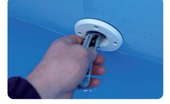
Now locate the faceplate and attach gasket for the inlet low level suction fitting.
