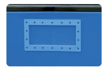
Carefully cut out the excess liner material from inside the skimmer faceplate to reveal the skimmer.
