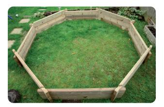
12 Fit the next layer of planks so each side has 2 layers.
