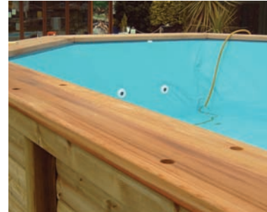
Once constructed, add in the liner and fill with water
