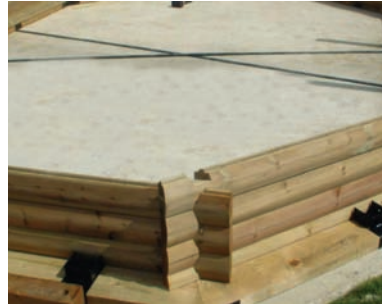
Lay out the base structure and start to build the wooden sections which fit together perfectly
