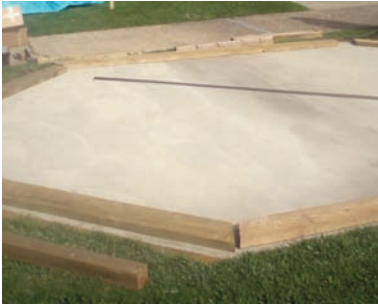
Concrete level base
