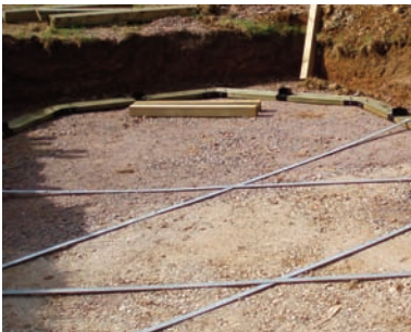
Dig the hole and prepare a flat base
