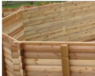
Build the wooden surround
